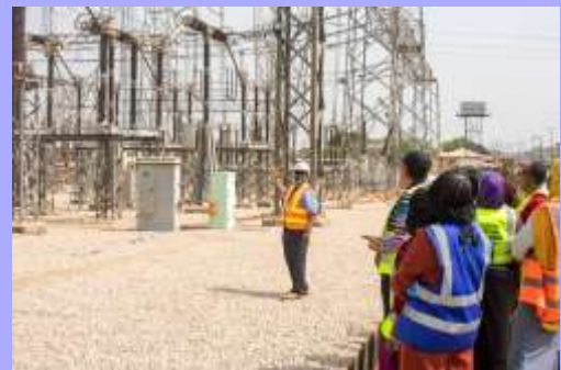
Engr. Omotosho of TCN taking APWEN Members in the Technical tour of the Facility.
